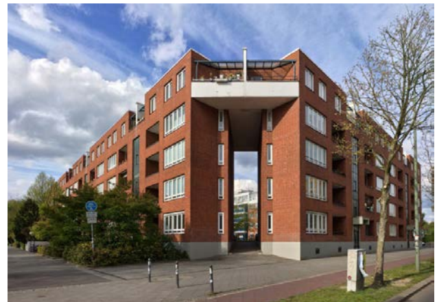
Figure 10. Residential building in Vinetaplatz, by Josef Paul Kleihues. © Gunnar Klack/flickr
