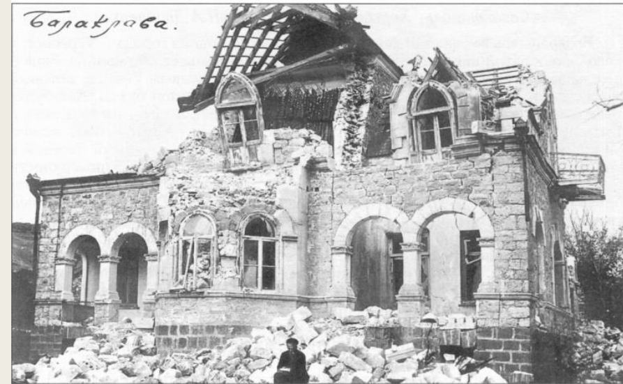
Fig.5. Destruction during the Crimean earthquakes of 1927: a – the Swallow's Nest castle, Alupka; b – residential building in Balaklava
