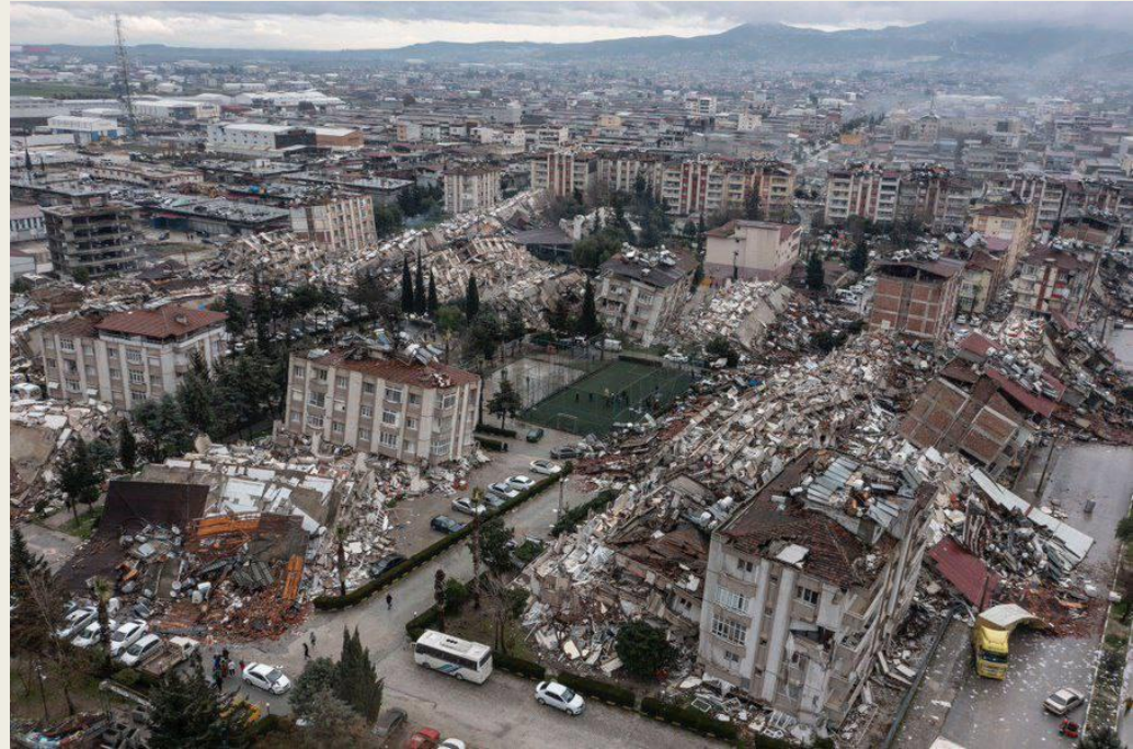
Fig. 6 Consequences of the earthquake in Hatay, Turkey. February 2023
