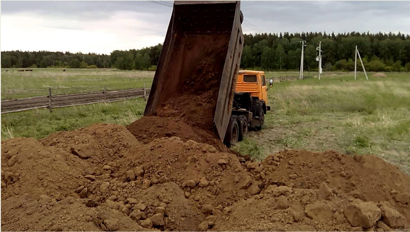
Fig. 2. Backfilling to increase the level of the territory
