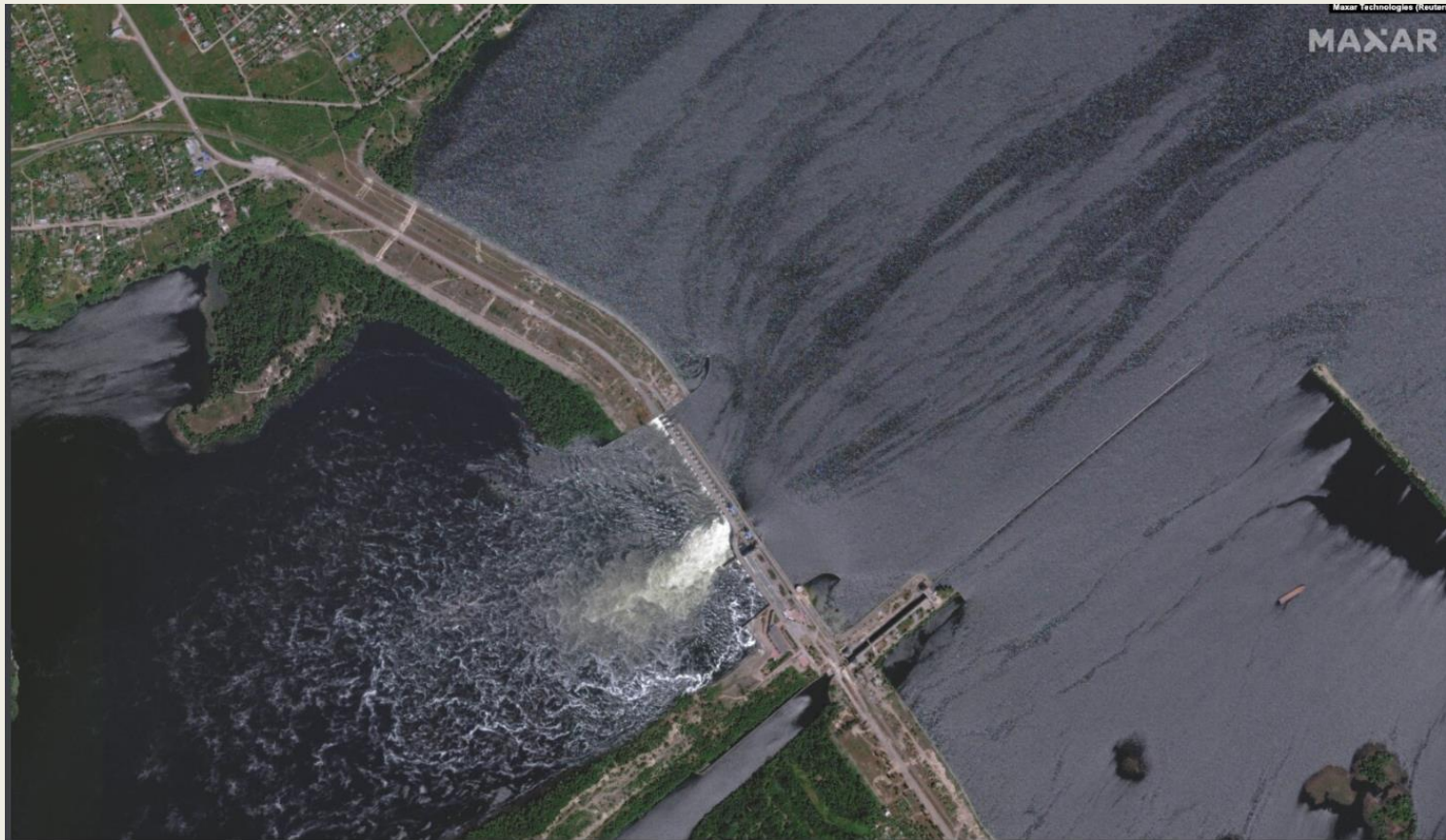
Fig. 8. On June 6, 2023, around 03:00 a.m., the Russian military blew up the dam of the Kakhovskaya Hydroelectric Power Station
