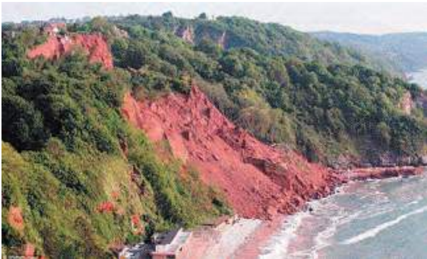
Fig. 3.9.2. Destruction of an apartment building as a result of a landslide caused by abrasion, Devonshire, England https://www.dailymail.co.uk/news/article-2337012/Cliff-cul-sac-Britains-dangerous-street-home-collapsed-sea-evacuated-safety-fears.html
