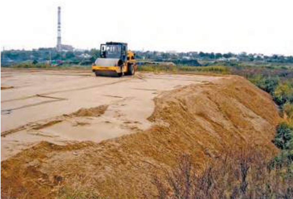
Fig. 4.7.2. Compaction of an embankment with a road vibratory roller https://www.geosisp.ru/typy-issleduemyh-gruntov/
