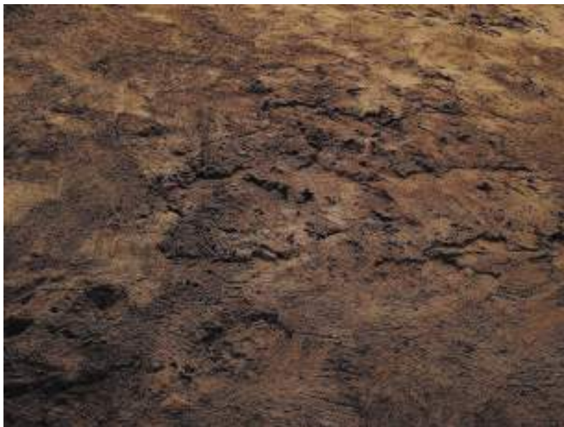
Fig 4.6.4. Swelling soil intact structure
