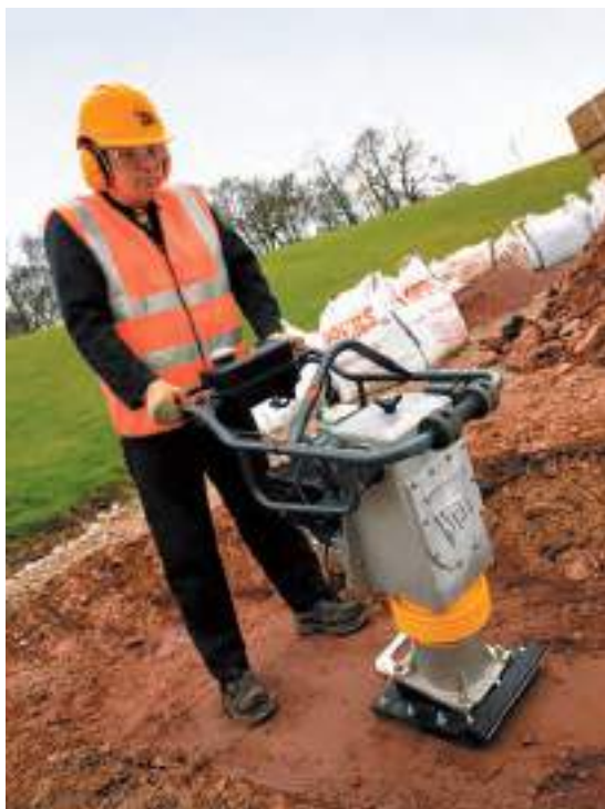
Fig 4.5.11. Compaction of subsidence soil with a hand vibrating compactor http://profmashine.ru/wp-content/uploads/2014/03/716550514.jpg
