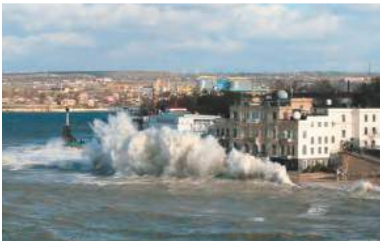
Fig. 3.9.13. Passive protection of the embankment by the wave-breaking wall in Sevastopol, Crimea http://ecodevice.com.ru/photogallery
