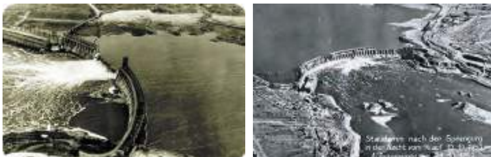
a b Fig. 3.13.5. Dam of the Dnieper hydroelectric station: a – after the explosion in 1941; b – 15.10.1943 г.
