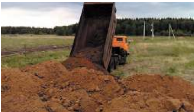
Fig. 3.12.2. Backfilling to increase the level of the territory http://megawood.pro/file/2015/11/29/vyravnivanie_1.jpg
