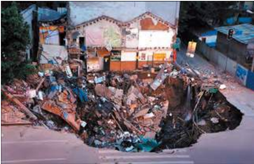
Fig. 3.11.4. Failure in the construction of subway in Guangzhou, China http://i.dailymail.co.uk/i/pix/2013/01/29/article-2270006-173AACAB000005DC-44_1024x615_large.jpg
