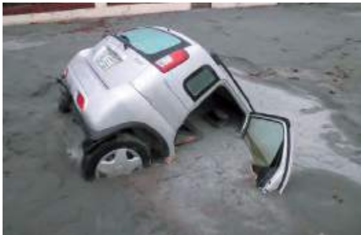
Fig. 3.10.19. Submersion of a car in liquefied sand, 22.02.2011, Christchurch, New Zealand http://www.maipark.com/assets/uploads/Erly.pdf
