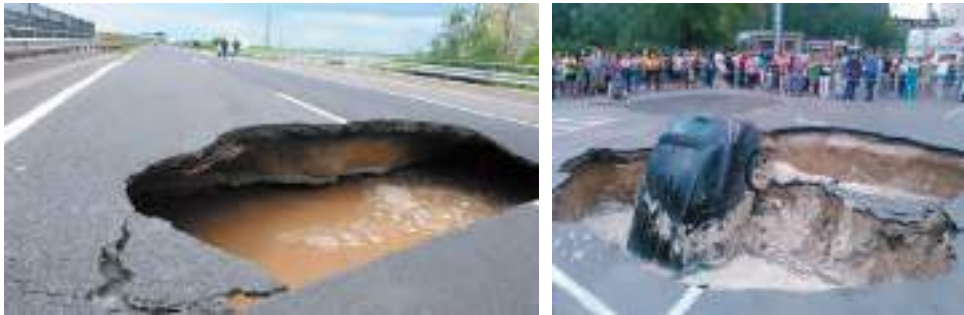
Fig. 3.1.6 a, b. Suffusion cavities due to groundwater ruptures
