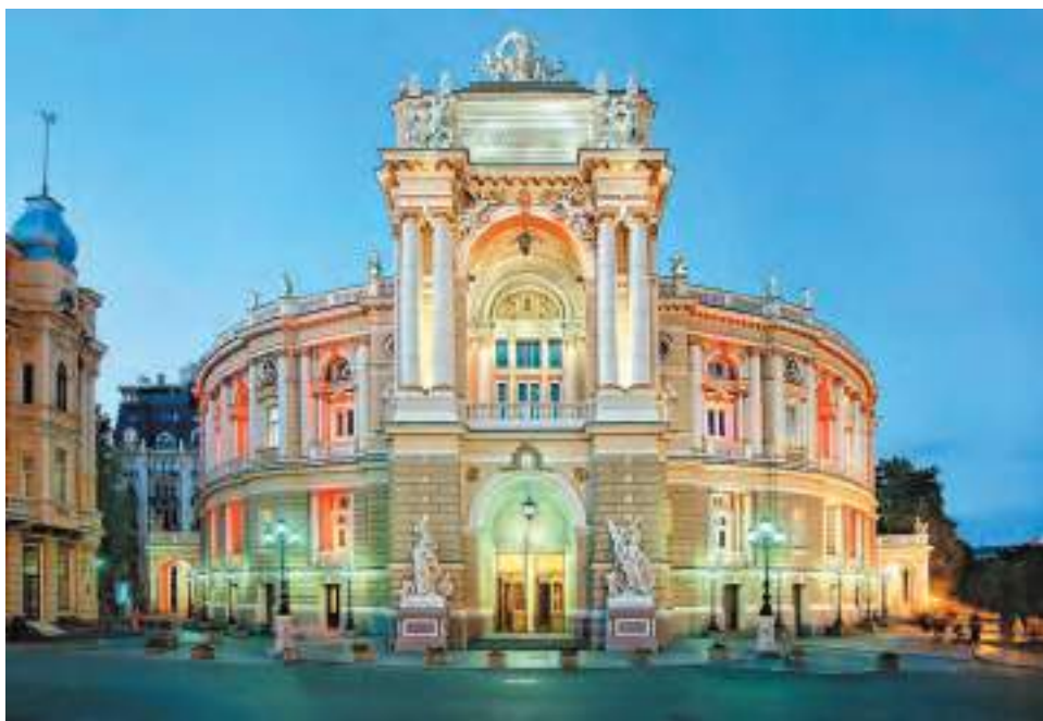
Fig. 4.5.15. Odessa Opera House, built on loess soils, fortified with silicatization http://www.tic.in.ua/wp-content/uploads/2015/09/1001.jpg
