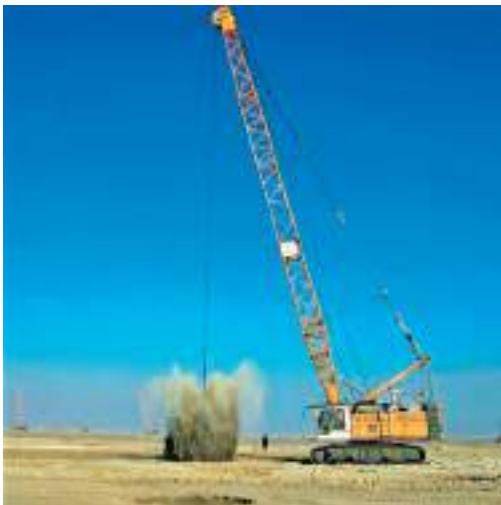
Fig. 4.7.5 a, b – Tamping soil on a grid in a checkerboard pattern
