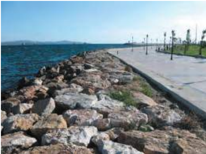
Fig. 3.9.12. Protecting the embankment with the help of stable laying of blocks in Bandirma, Sea of Marmara, Turkey. Photo by V. Iegupov
