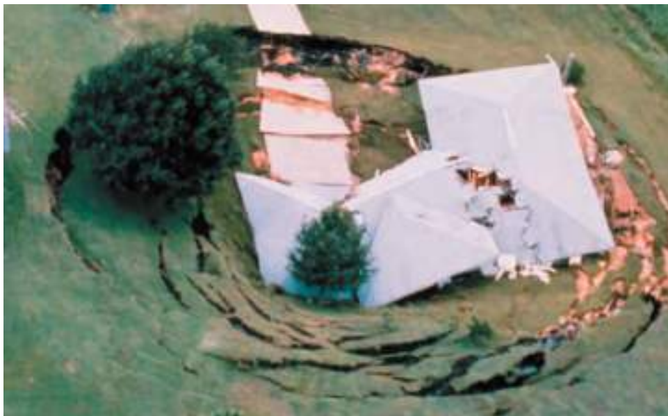
Fig. 3.11.1. Destruction of buildings during the subsidence of the earth's surface in the form of a trough
