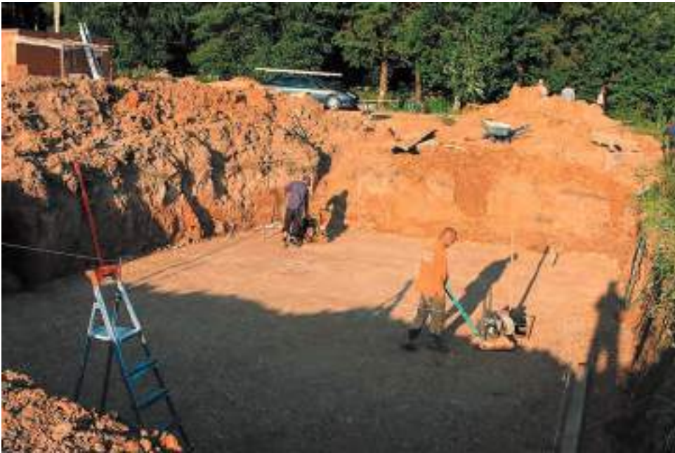
Fig. 4.7.1. Compaction of subsiding soil at the bottom of the pit with manual vibration methods http://stroidom-mozhaisk.ru/photo/stroy_proc/011.jpg
