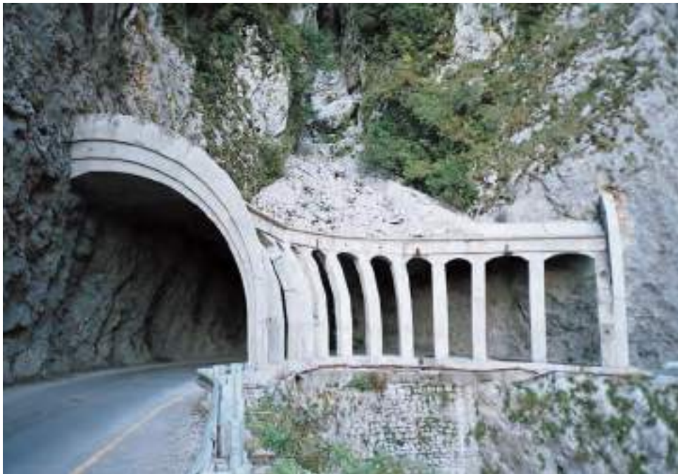
Fig. 3.3.15. Protective anti-rockfalling gallery http://otktravels.narod.ru/travels/more2/more2_38.htm
