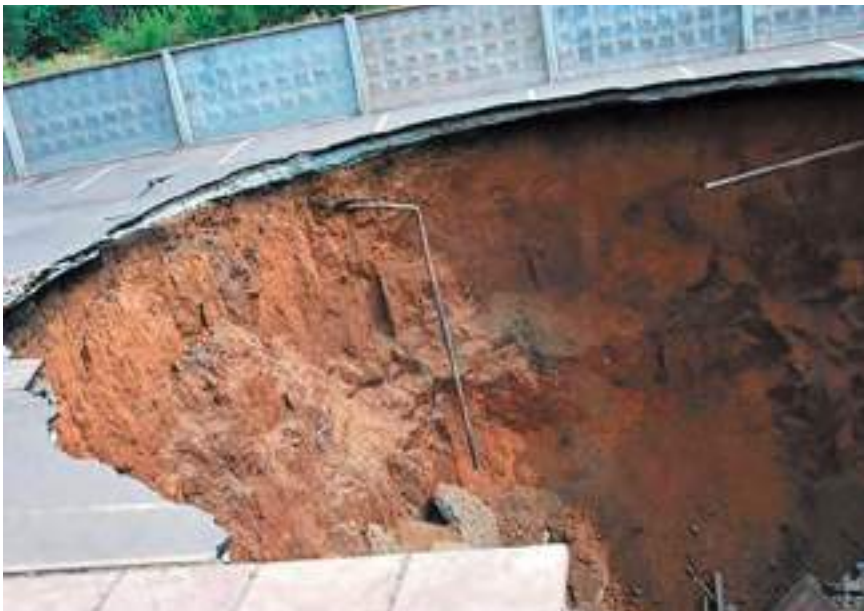
Fig. 3.11.5. Failure in the mined-out space during iron ore mining (the central market of the city of Kriviy Rig) https://encrypted-tbn2.gstatic.com/images?q=tbn:ANd9GcQK5VKidl73zwhmGq8JUrmkSpDIHHVHlPX9TOU84w3FtP5e0Xn
