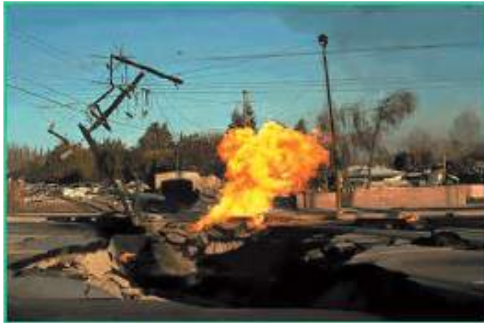
Fig. 3.10.18. Pipeline rush during lateral spreading, Northridge, USA, 1994 http://www.maipark.com/assets/uploads/Erly.pdf
