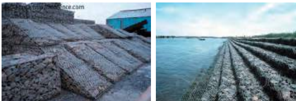
Fig. 3.8.13. Designs to strengthen the coast: a – gabions of various shapes
