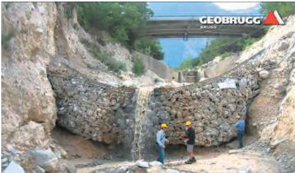
Fig 3.5.4. Gabion Type Mudguard Dam
