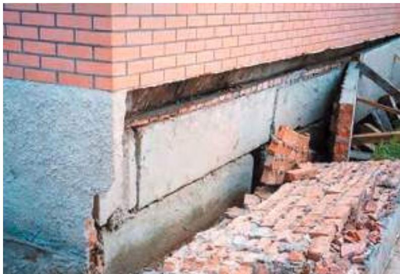
Fig. 4.5.8. Destruction of the foundation during the subsidence of the underlying loess strata http://www.ua.all.biz/img/ua/service_catalog/567991.jpg
