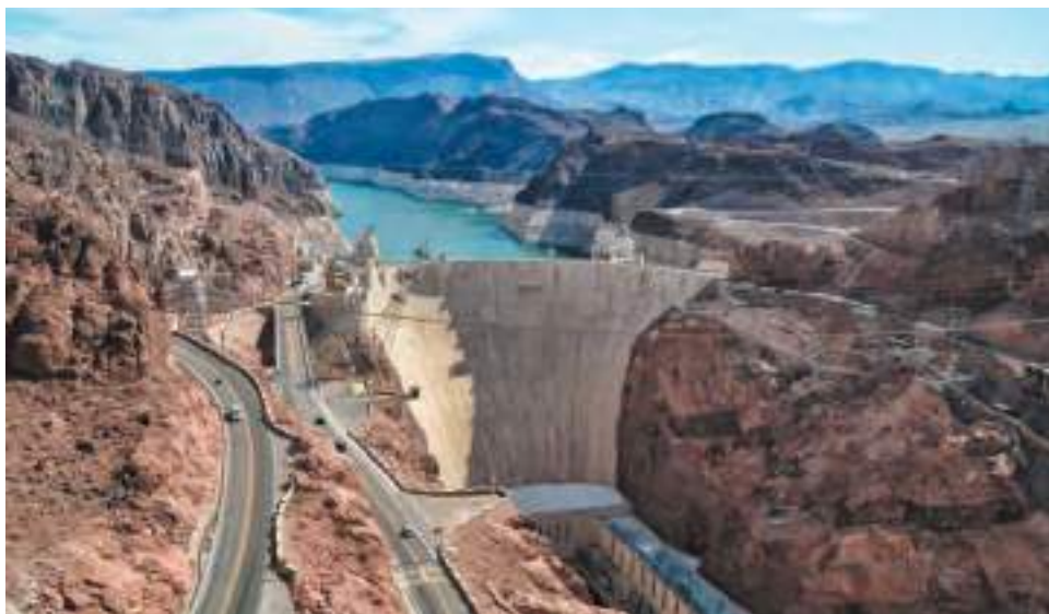
Fig. 2.3.12. Lake Mead Reservoir and Hoover Dam (221 m high) on the Colorado River, the border of Arizona and Nevada, USA. The creation of a reservoir led to the transformation of the surrounding area into an area of increased seismicity Photo by Iu. Egupov
