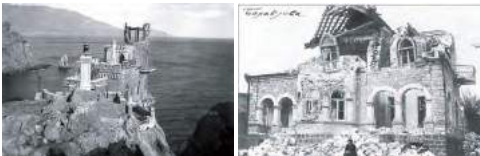
a b Fig. 2.3.5. Destruction during the Crimean earthquakes of 1927: a – the Swallow’s Nest castle, Alupka http://журналкрым.рф/uploads/posts/2015-07/1438185678_ lastochkono-gnezdo-posle-zemletreseniya-1927-goda.jpg ; b – residential building in Balaclava http://www.krimoved-library.ru/images/ka2002/1-45.jpg
