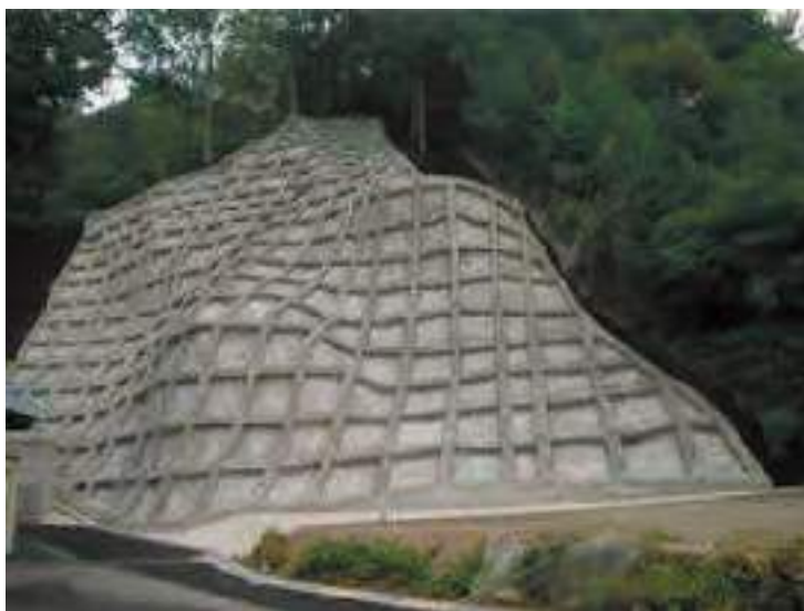
Fig 5.3.6. Example of Spray Crib works (source: JET)
