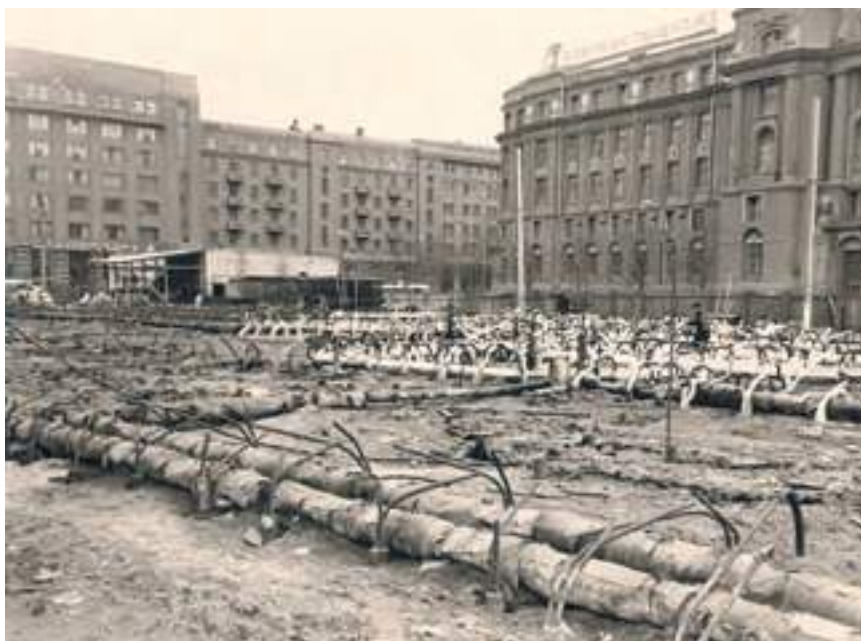
Fig. 3.10.12. Freezing quicksand soils during the construction of the metro station “Yuzhny Vokzal” in Kharkov (1971) http://www.ljplus.ru/img3/e/m/ems_viking/stroit_20yagni.jpg
