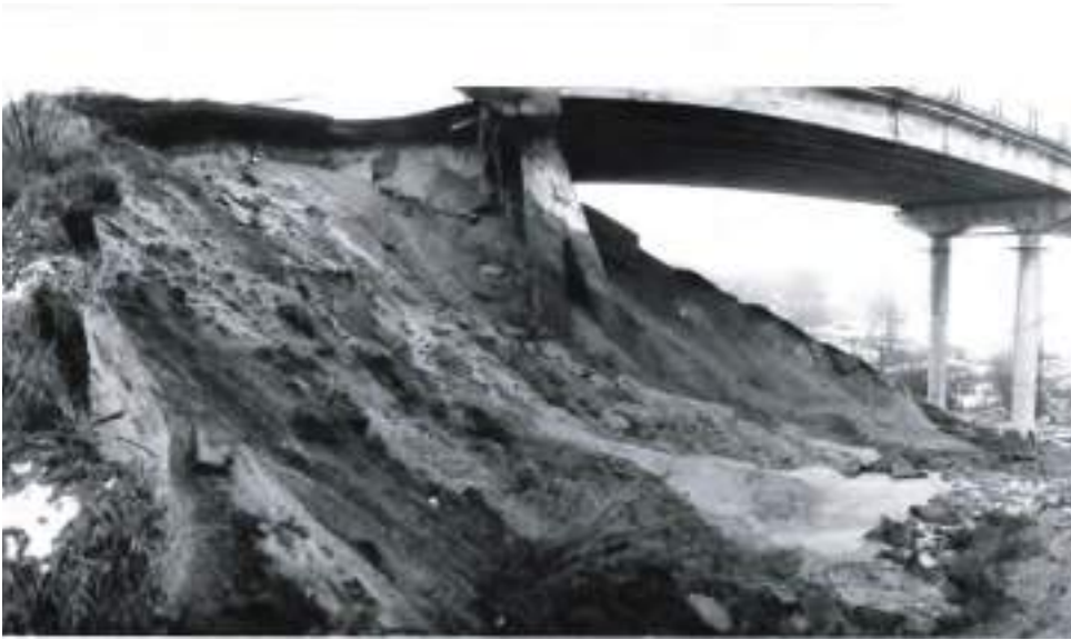
Fig. 3.4.11. Modern landslide on an artificial dam, Kharkiv, Ukraine Photo by G. Strizhelchik
