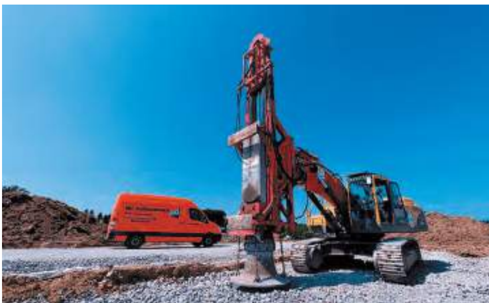
Fig. 4.7.3. Dynamic self-propelled rammer compacts the soil base
