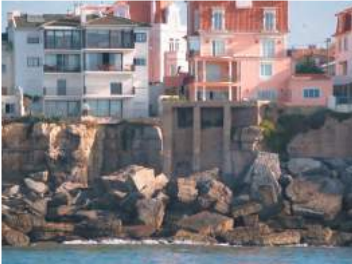
Fig. 3.9.11. Coastal protection using rock boulders in Estoril coast, Portugal https://geologicalintroduction.baffl.co.uk/?p=183
