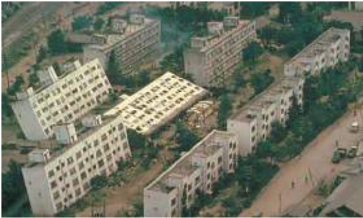
Fig. 3.10.16. Destruction of residential buildings during liquefaction of soil 16.06.1964, Niigata, Japan http: //learnlearn.net/verdensrommet,jorda/Vannb.htm
