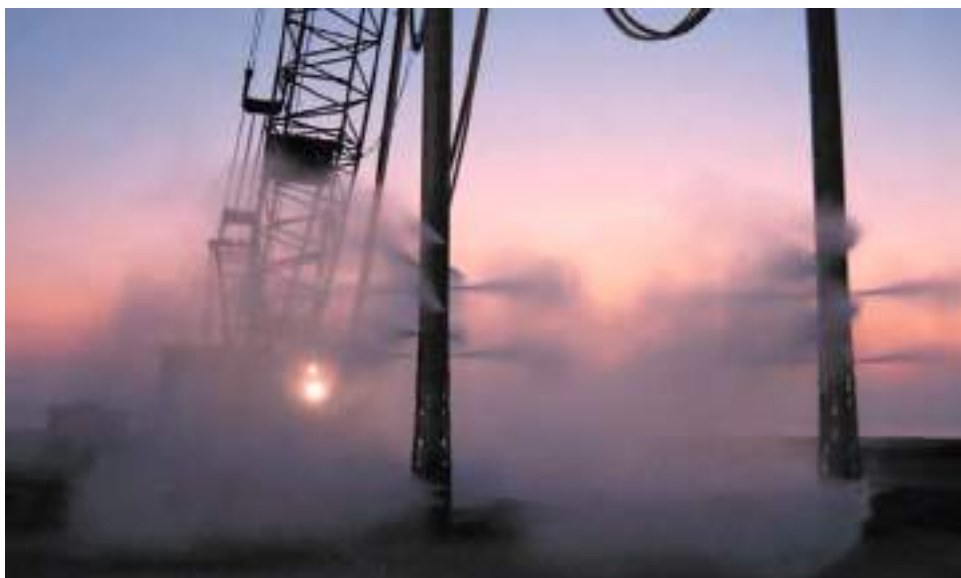
Fig. 4.7.7. Deep vibration compaction of soil: a – submersible cone; b, c – water supply through nozzles in the working body http://www.menard-russia.ru/images/heavy-tamping-slider-5.png
