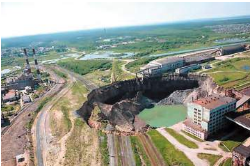
Fig. 3.2.17. Technological karst failure in Berezniki, Russia, which occurred in December 2011. Since then, the funnel has swallowed up several industrial buildings of the mine-building department http://earth-chronicles.ru/news/2014-07-25-68765
