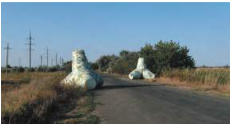
Fig. 3.9.14. Tetrapods are one of the most effective structures for shore protection structures. Photo by V. Iegupov
