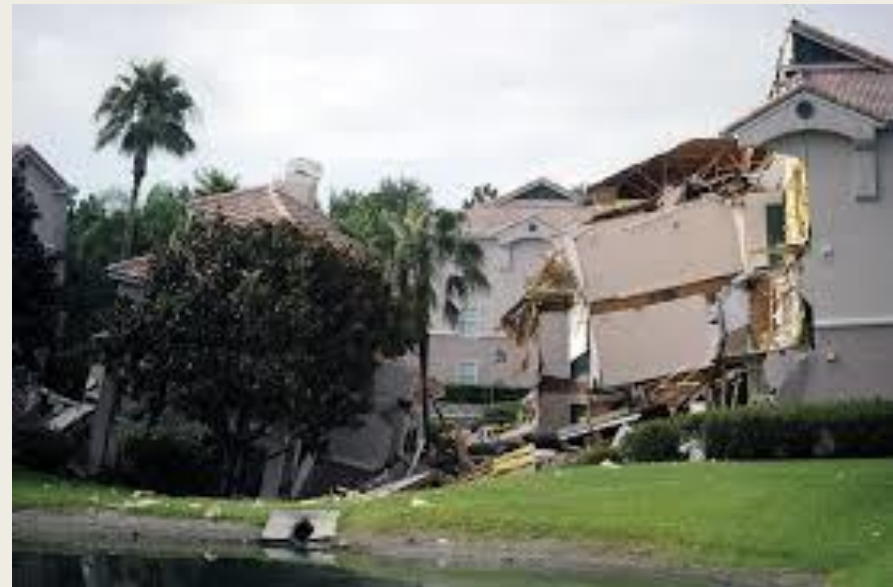
Fig. 19. Karst sinkholes: a - failure under the tram track, Nizhny Novgorod Region; b - failure on the territory of summer cottages, Solikamsk; c - part of the hotel collapsed into a large sinkhole in Clermont, Florida, USA
