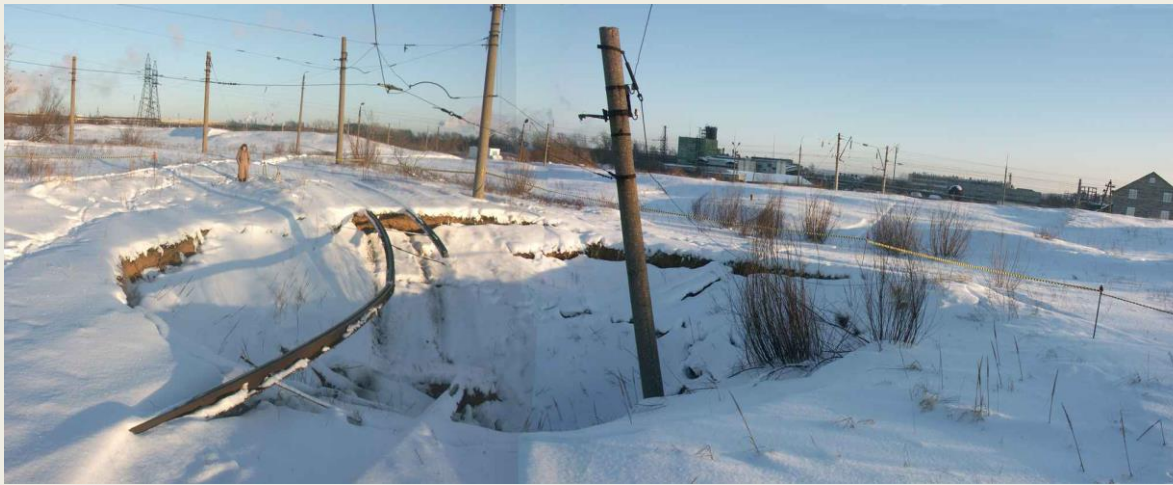
Fig. 19. Karst sinkholes: a - failure under the tram track, Nizhny Novgorod Region; b - failure on the territory of summer cottages, Solikamsk; c - part of the hotel collapsed into a large sinkhole in Clermont, Florida, USA
