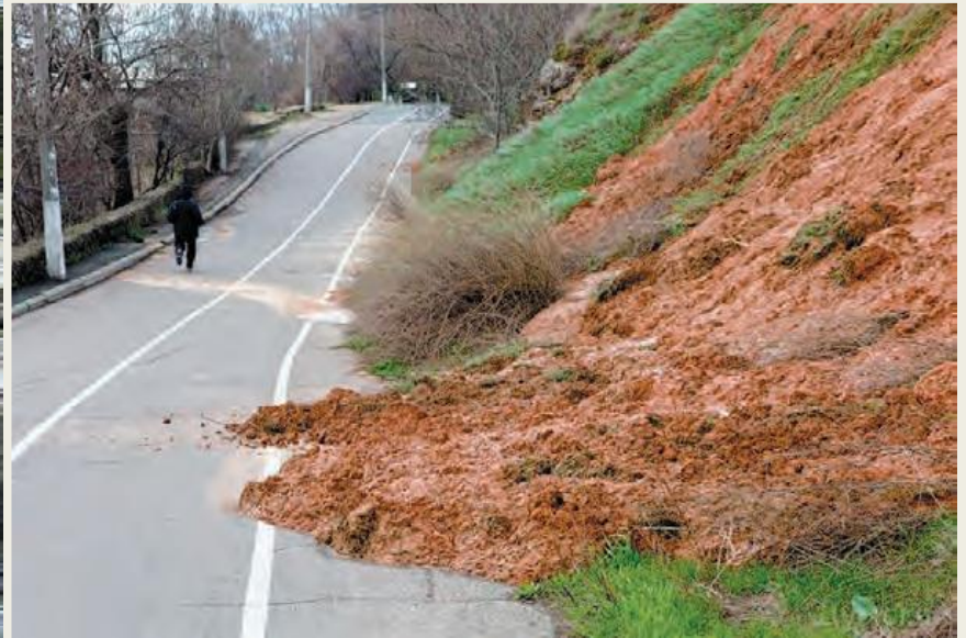
Fig. 16. Sweeping of a slope composed of loesslike loams
