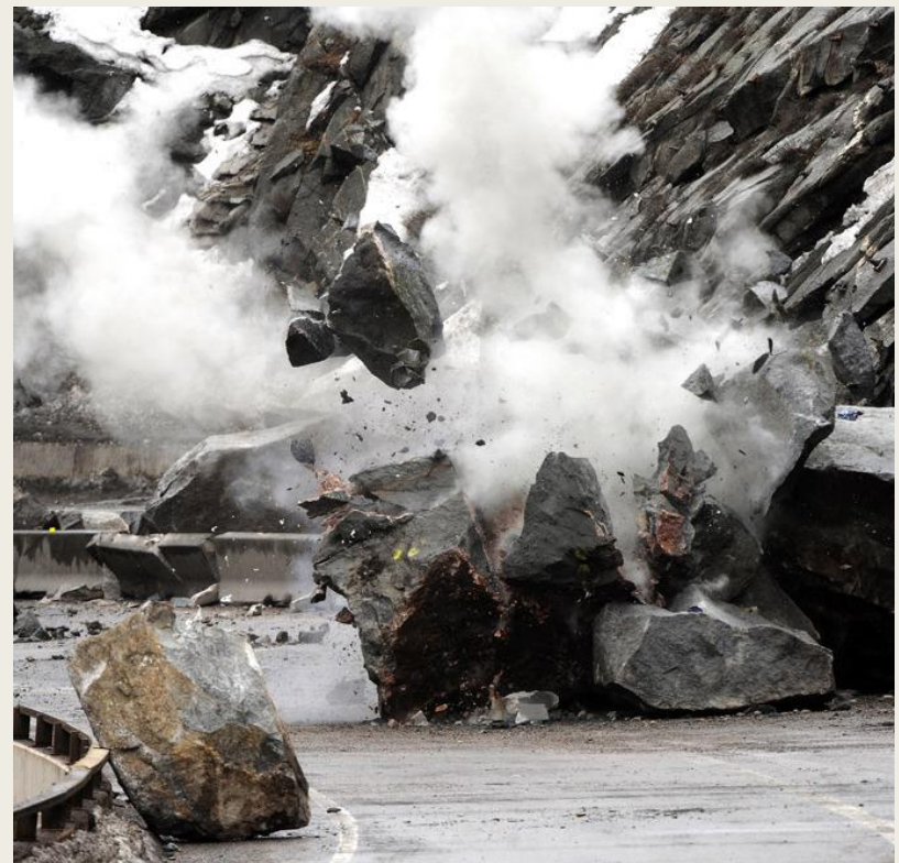
Fig.11 Collapse of blocks on highways in the mountains: Colorado, USA;
