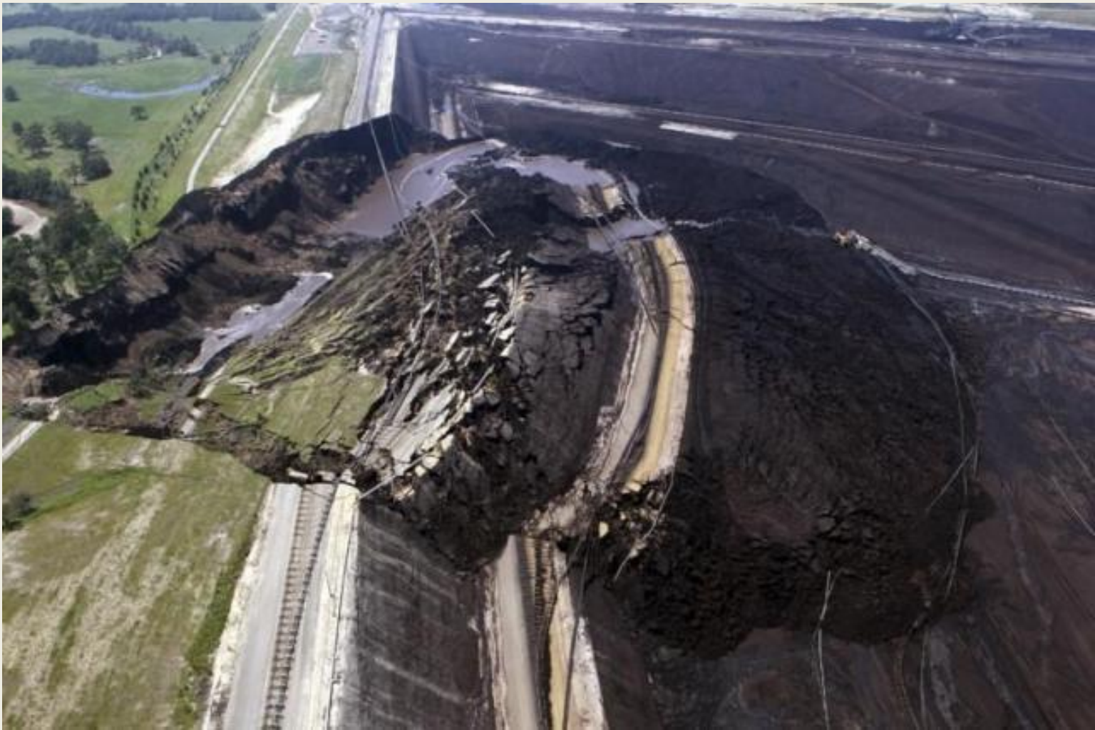
Fig. 25 Landslide Terraces, Groundwater Outcrops
