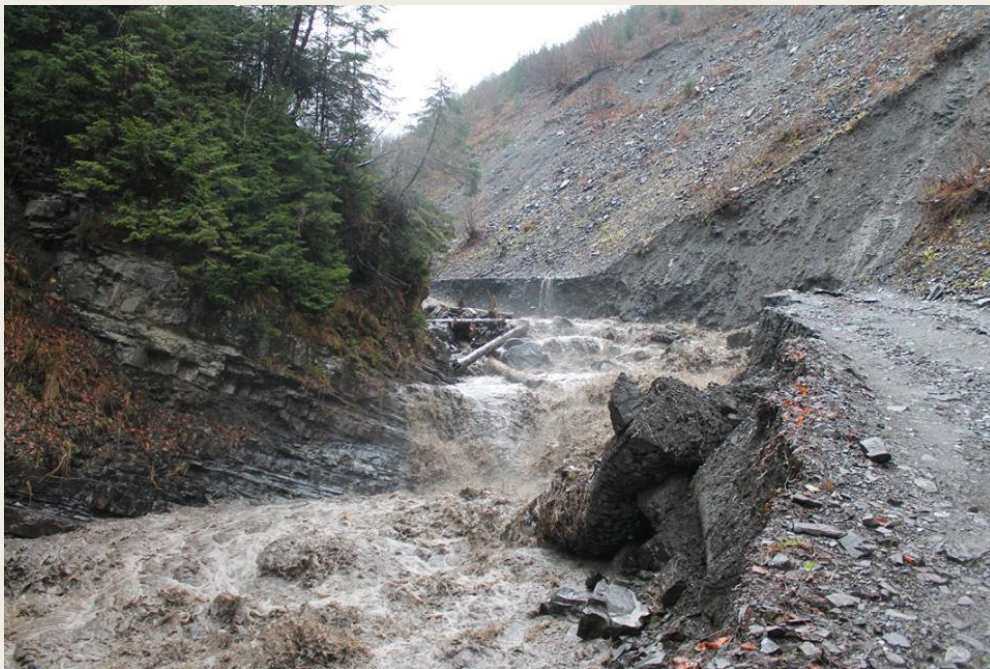
Fig. 36 a – the road washed out by mudflow in the Carpathians; b, c – the consequences of mudflows
