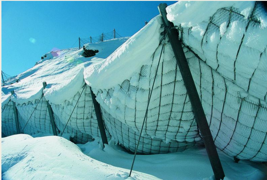
Fig. 43. Snow retention nets
