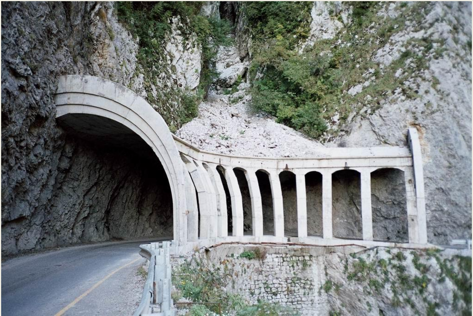
Fig. 13 Protective anti-rockfalling gallery
