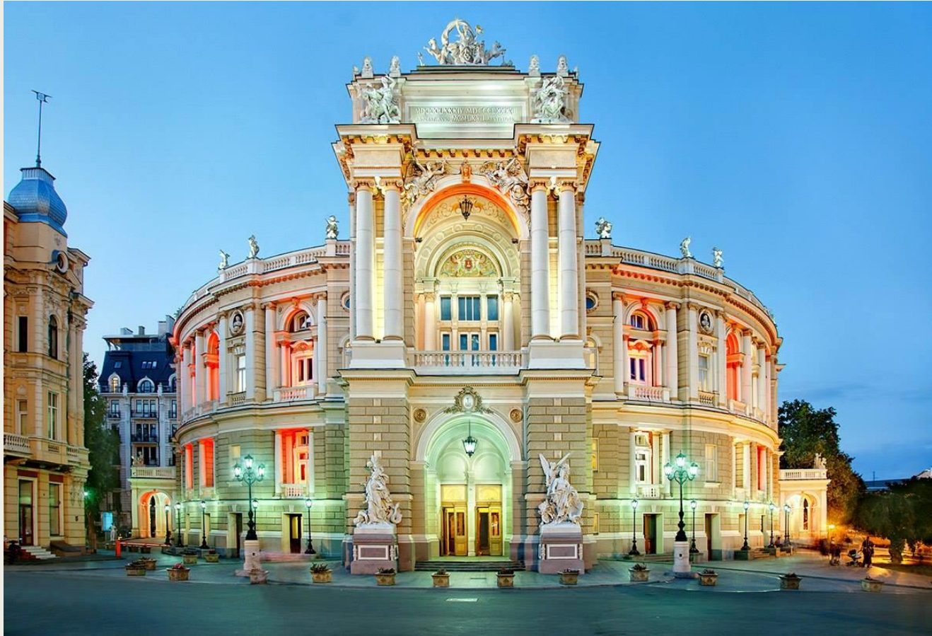
Odessa Opera House, built on loess soils, fortified with silicatization
