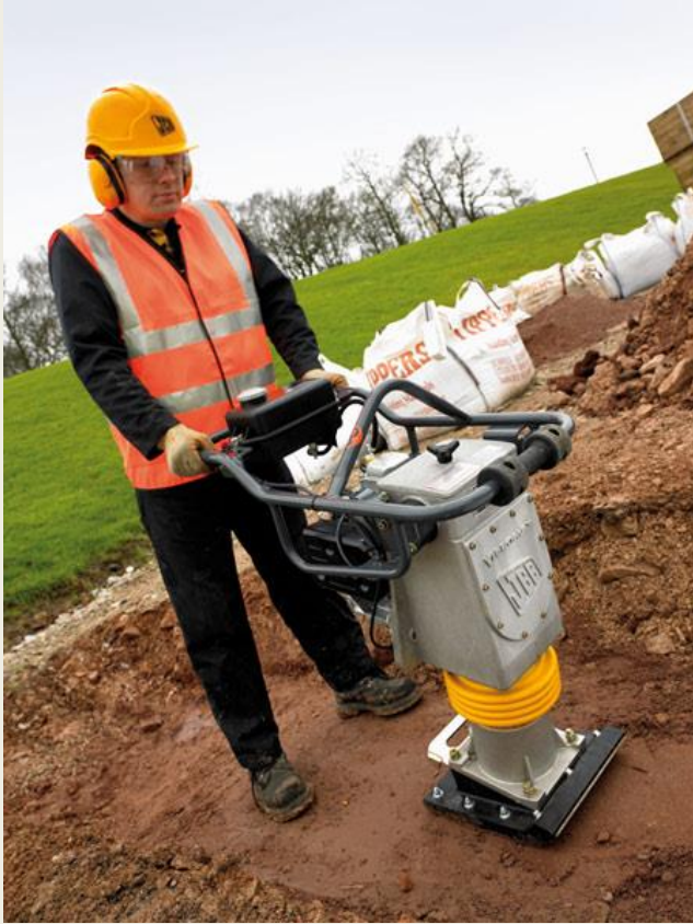
Compaction of subsidence soil with a hand vibrating compactor
